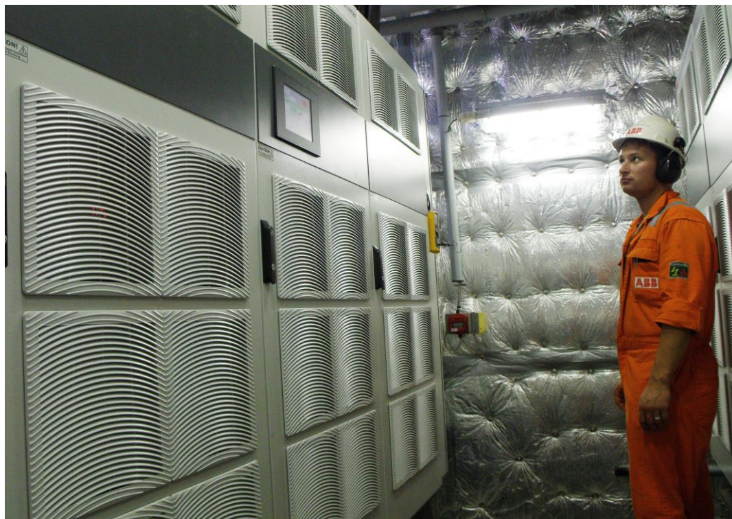
2 x 1700kVA @45°C PCS100 SFC onboard installation, FPSO
