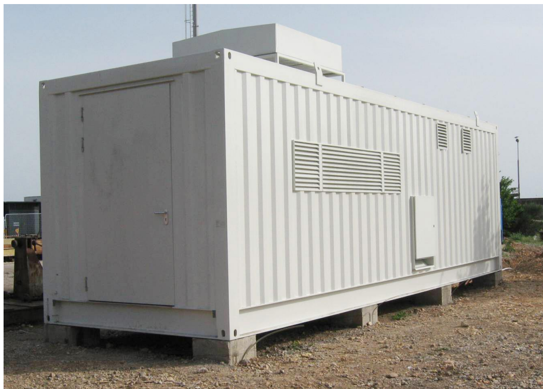
2 x 1250kVA PCS100 SFC containerised
