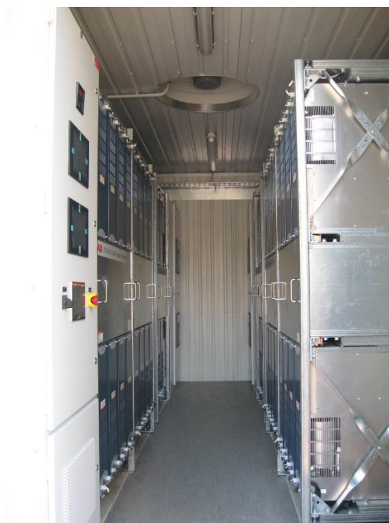
PCS100-03-10E-B35 & PCS100-03-10E-B36 integrated into container solution
