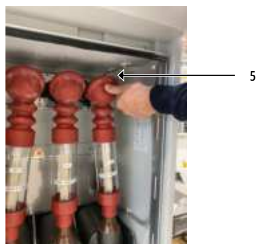
Figure 4-27: Unlock fuse holder
