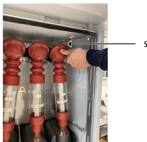
Figure 4-27: Unlock fuse holder
