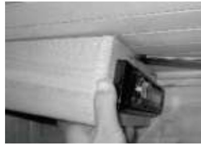
FIG-17 Screwing in the Radio Wood Housing
