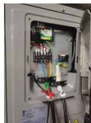
2. Slide the panel down to release the clips and pull away.
