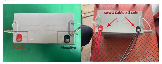
b. Find the positive and negative poles of the inverter input terminals, install the cables and tighten them. Red: positive, black: negative.
