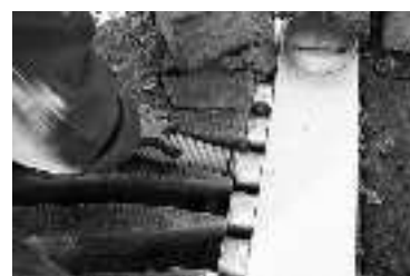
Manifold in floor insulating material before casting
