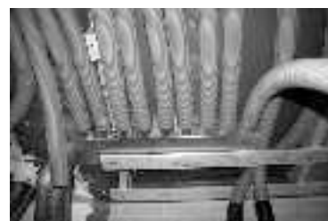
Manifold beneath ceiling inside climate shield
