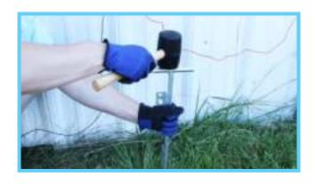
Insert the ground rod into the soil within a 20 foot radius of your energizer
