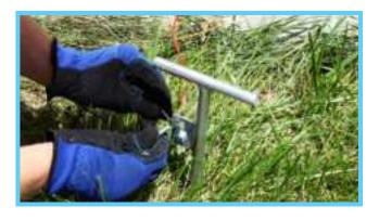
Attach the negative jumper clip to your ground rod.
