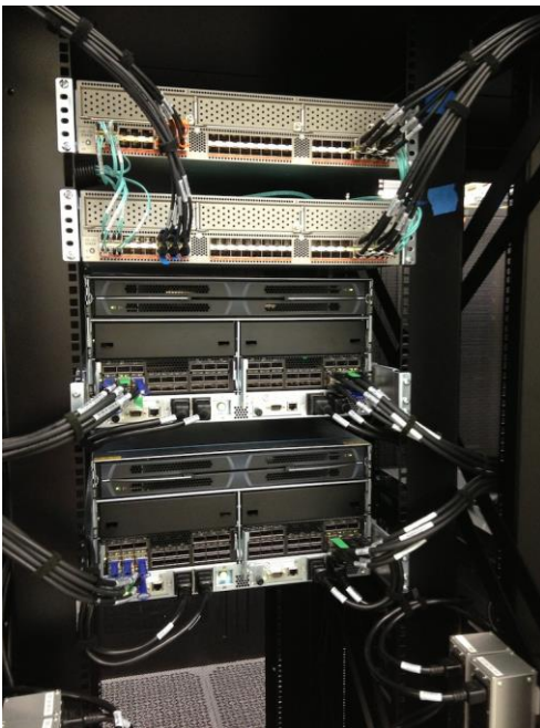
Figure 7: Cluster Front and Back-end Switches (Rack F Above)
