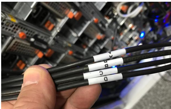
Figure 10: Network Cable Labeling Example
