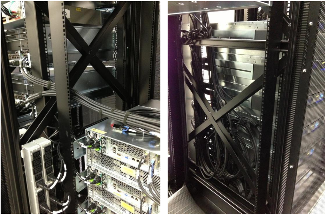
Figure 8: Rear and Side views of Rack Showing Mailbox Space and Backend Network Cabling (Rack E Above)
