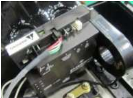
Figure 2: CoreSense Diagnostics sensor module located in terminal box
