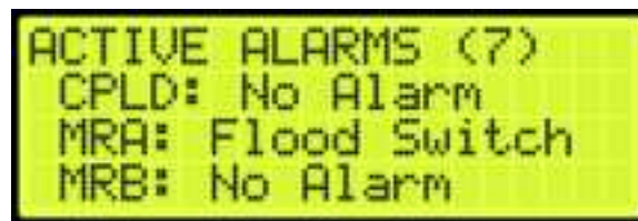
Figure 756: Active Alarms Menu
