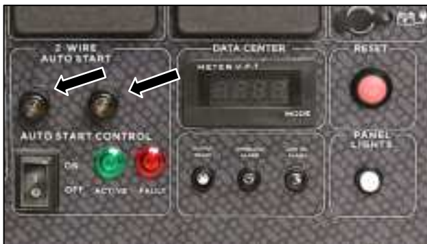
Figure 13 2-Wire Auto Start Panel
