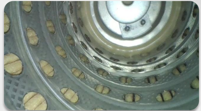
Lubrication Filter Inspection Using a 3.9mm VQ2 039 1500 4
