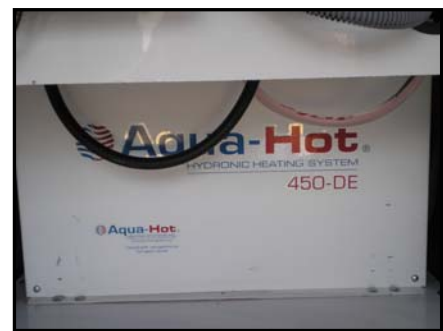
Figure 3-2. Hydraunic Heating System
