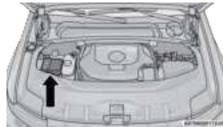
Power Distribution Center
