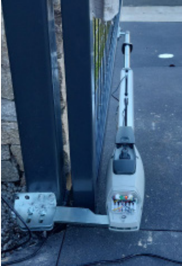
Incorrect setup showing the arm running parallel with the gate
