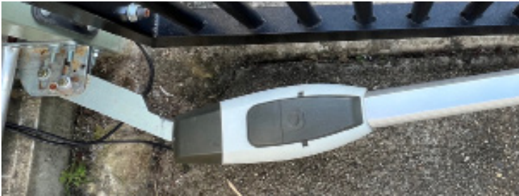
Correct setup showing the arm with an angle to the gate
