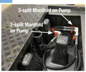
Check These Pump Assemblies should be under the Pump Access, and the PVC Center Support Column should be in the center of the basin.
