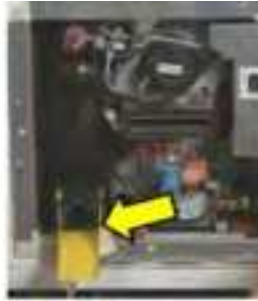
Draining the Aqua Go Water Heater
