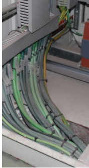
Figure 2 – Yellow and Green cable for earthing.
