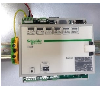
Figure 4 – Example of earthing for EMC.
