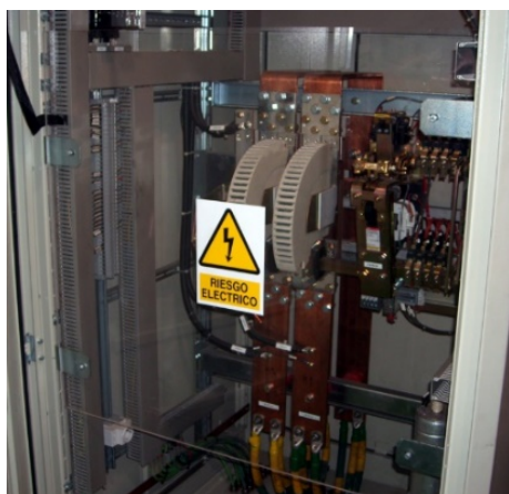
Figure 1 - Barrier of protection for elements with high voltages.
