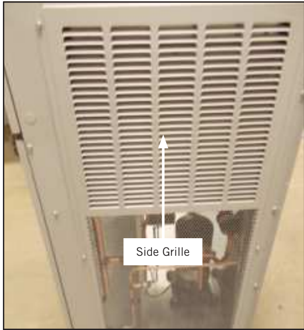
FIGURE 2 Remove Side Grilles
