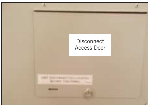
FIGURE 1 Disconnect Power
