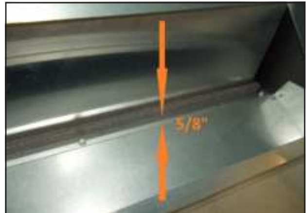
FIGURE 7 Install Exhaust Blade Assembly
