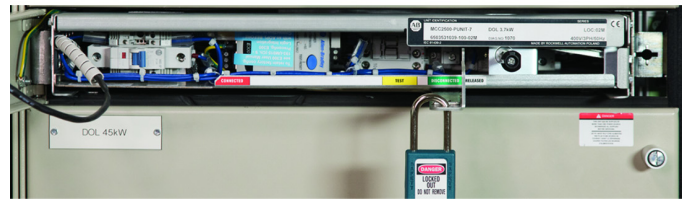
Withdraw lever in the Disconnected position (and locked out).
