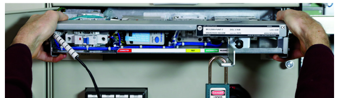
Withdraw lever in the Released position (and locked out).
