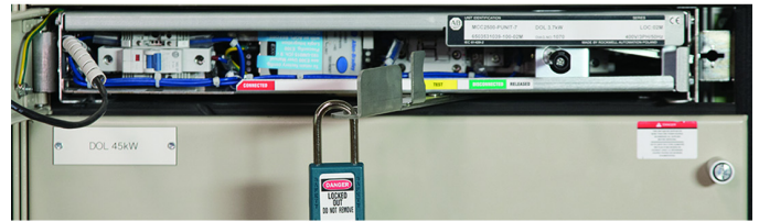
Withdraw lever in the Test position (and locked out).
