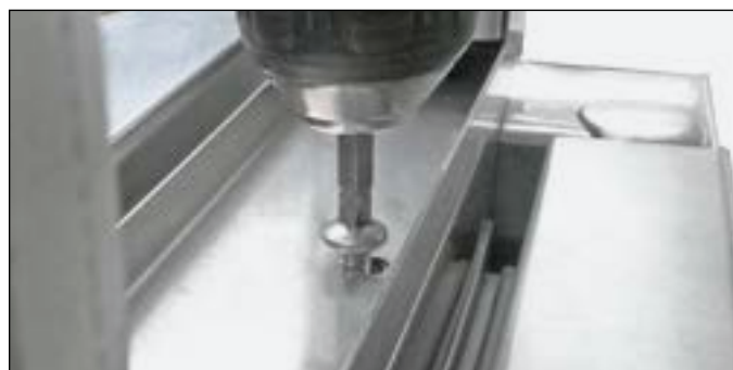
FIG. 10. Remove the screws from the metal channel.
