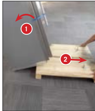
FIG. 10B. Then, tilt the unit backward and remove the skid.
