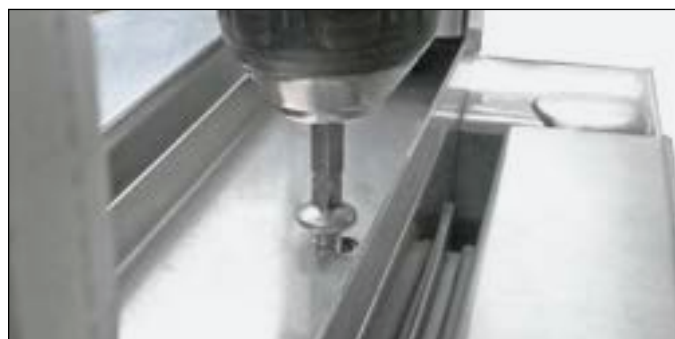
FIG. 10. Remove the screws from the metal channel.
