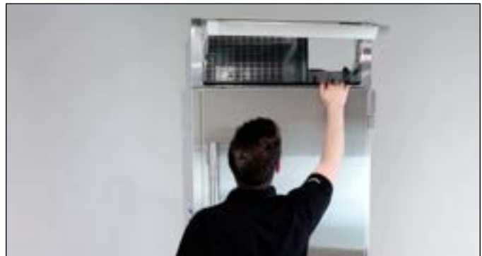
FIG. 3. Be sure to inspect the rainshield.
