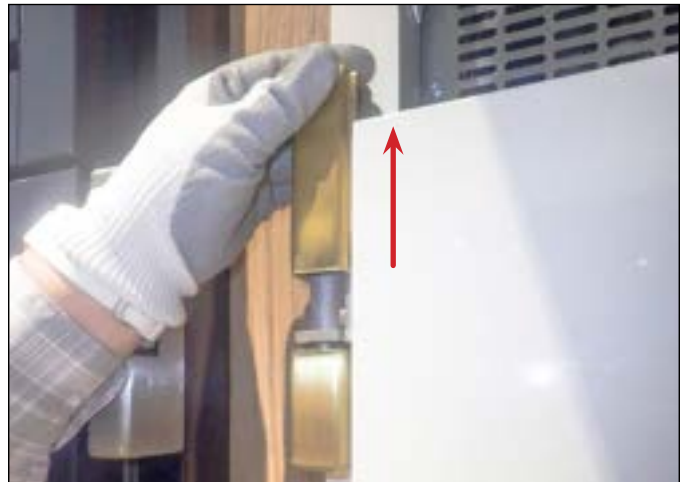
FIG. 2. Remove the hinge covers.
