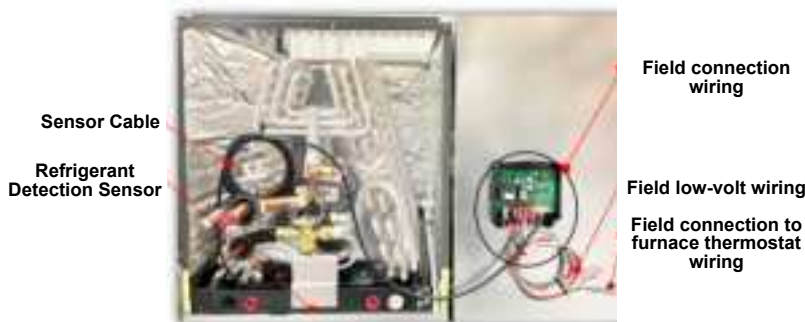
Figure A1 - Mitigation Control Boards (cover removed to show internal components)
