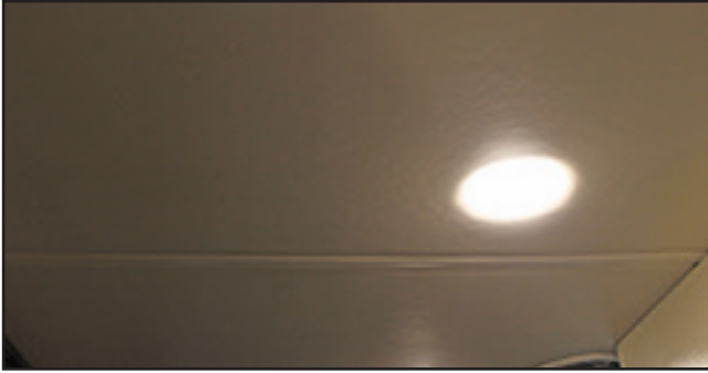
Figure 12-3: Typical ceiling in the Allegro Breeze
