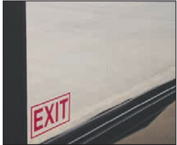
Figure 2-9: Emergency exit window
