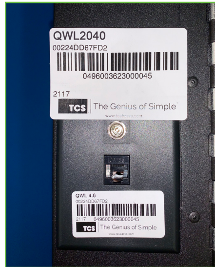
Placement of replacement Gateway label
