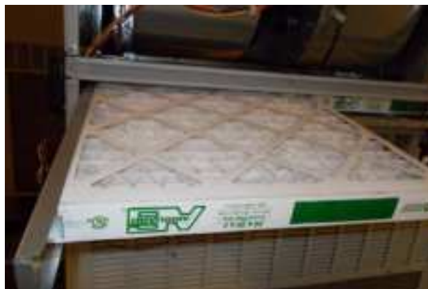
FIGURE 42 Install Left 2" Filter
