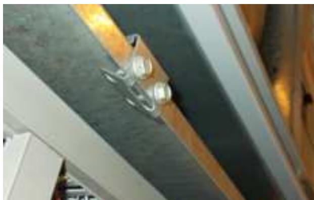
FIGURE 40 Re-Install Screws and Bend Tabs Up
