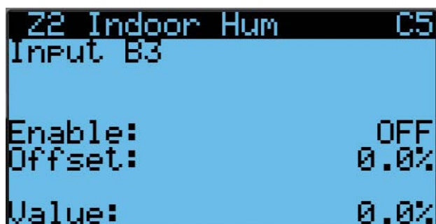
FIGURE 34 Enable/Disable Zone 2 Indoor Humidity Sensor
