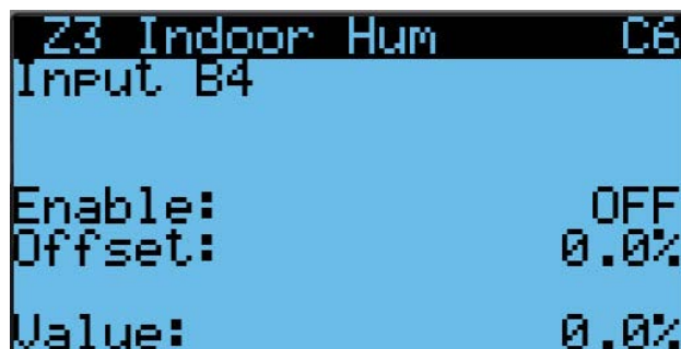
FIGURE 35 Enable/Disable Zone 3 Indoor Humidity Sensor
