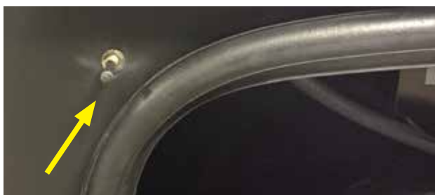
Fuel Pump Safety Lock-out Switch
