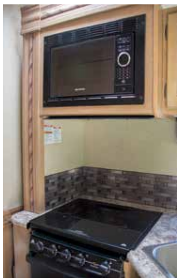
Typical range and microwave
