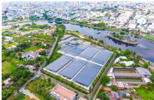
1.4 MW PV Plant Vietnam 🇻🇳
