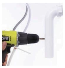
2. Choose where the drain clamp will be installed and drill a ¼inch. hole. The foam padding to the inside of the Drain clamp, around the hole.
