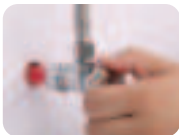
Shut off the water supply
