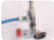
Valve installation complete
