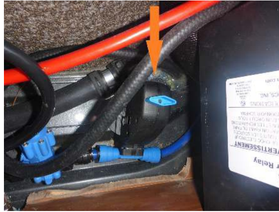
Alde front control valve in operating position
