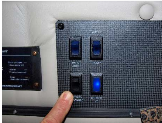
Battery disconnect switch
