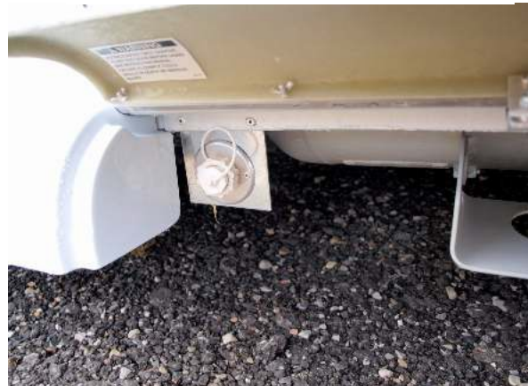
City water connection, driver's side behind front access bay door
