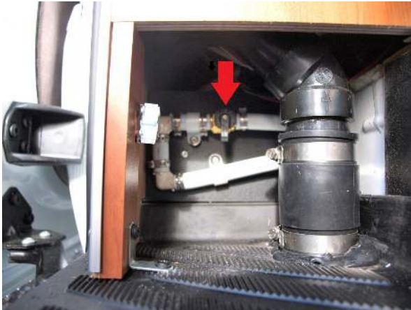
City water valve, shown closed (water is taken from on board)
