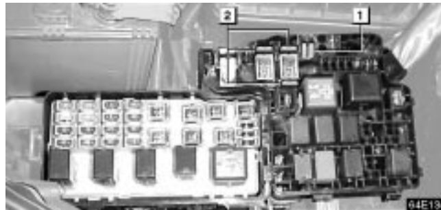
► Engine compartment 1 Pull-out tool 2 Spare fuses
