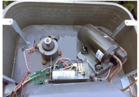
Picture 11: Early Mach 8 (style 1) with capacitors inside electric box
