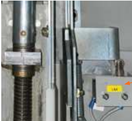
Figure 3: Racking mechanism with LS4 position switch shown
