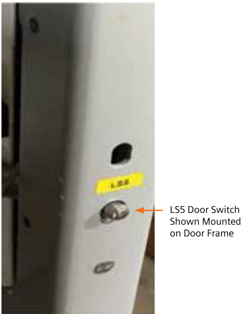
Figure 16 : LS5 Switch for GM-SG NonAR Compartment Door Shown
