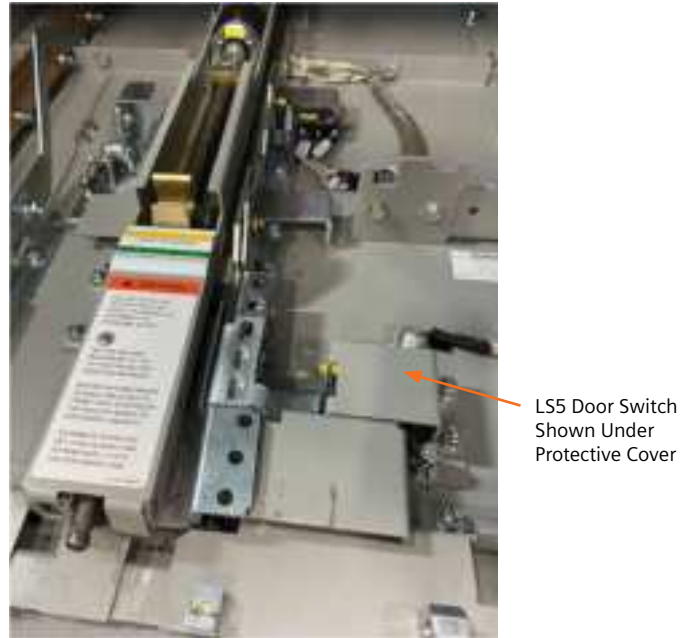
Figure 17: LS5 door Switch for GM-SG-AR Compartment
