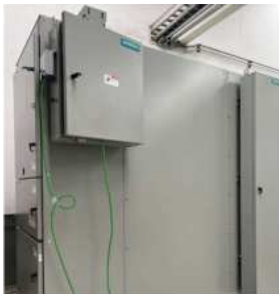
Figure 19: Local HMI Smart Setup with Control Cabinet Installed on the Side of Lineup
