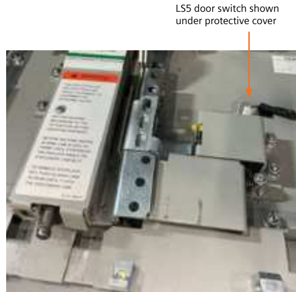
Figure 5: LS5 switch for GM-SG-AR compartment door shown
