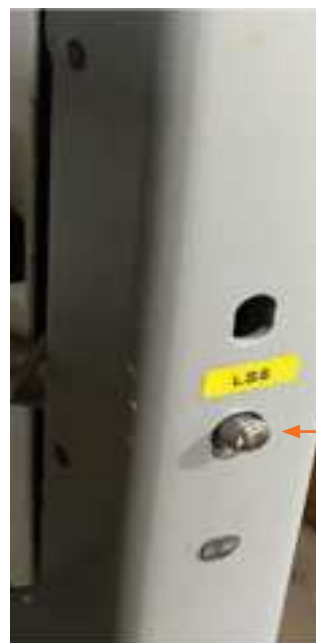
Figure 4: LS5 switch for GM-SG NonAR compartment door shown
