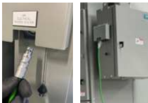
Figure 25: Port for PROFINET Cable Located in Front Side of SIERS Control Cabinet
