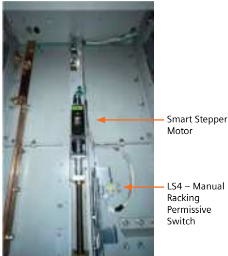
Figure 15: Racking Mechanism for HMI Setup
