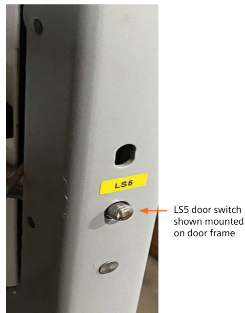
Figure 4: LS5 switch for GM-SG NonAR compartment door shown
