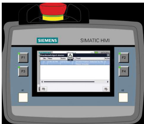
Figure 23: HMI Shown with Alarm Log
