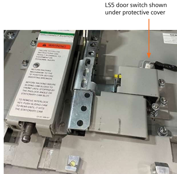
Figure 5: LS5 switch for GM-SG-AR compartment door shown
