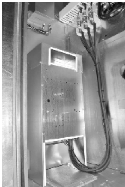
Figure 25 - Back View of Utility Entry and Power Switch from Control Compartment (70-140 ton Units)
