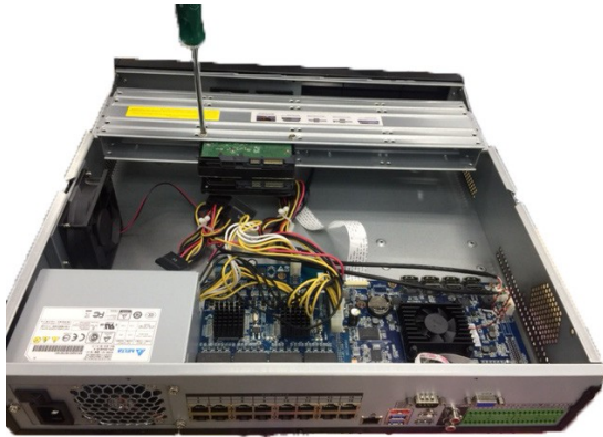
Figure 15-15 Placing the HDD
