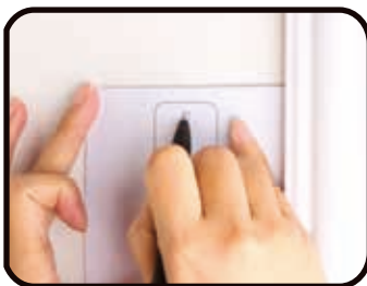
2.Mark the holes position of the lower and upper brackets as the left guide with a pen and keep in a vertical direction.
