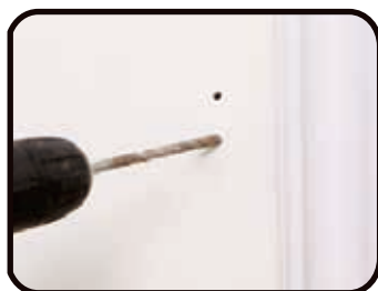
4.Drill holes with an electric drill as the marks
