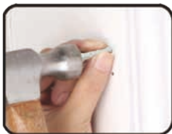
5.Insert the expansion screws to all holes
