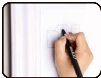
3.Mark the holes position of the lower and upper latches as the right guide with a pen.
