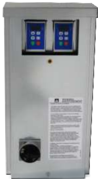
VFD KEYPADS IN E-BOX
