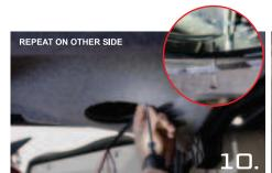
You can place a screw into the mount to mark the location of the hole
