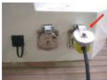
Shore power socket 220V - 32A (Reference 1)
