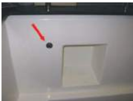
Drainage pump control - Shower
