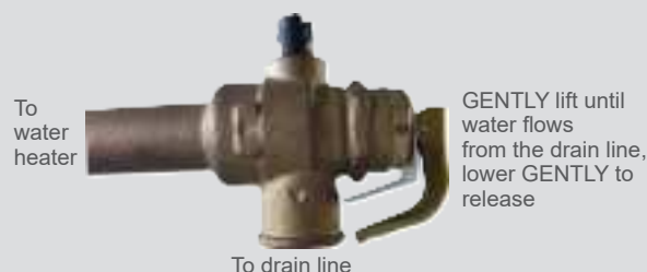
How to operate the easing gear
