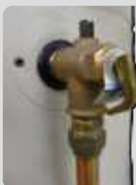
TPR position - top of cylinder
