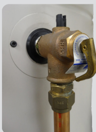
TPR position - top of cylinder
