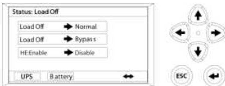
Figure 39. Typical system control screen
