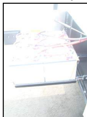
Figure 7-6. Batteries on Slide Tray
