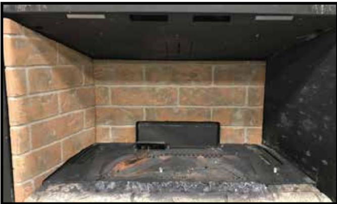
Figure 5 Left Refractory Installed
