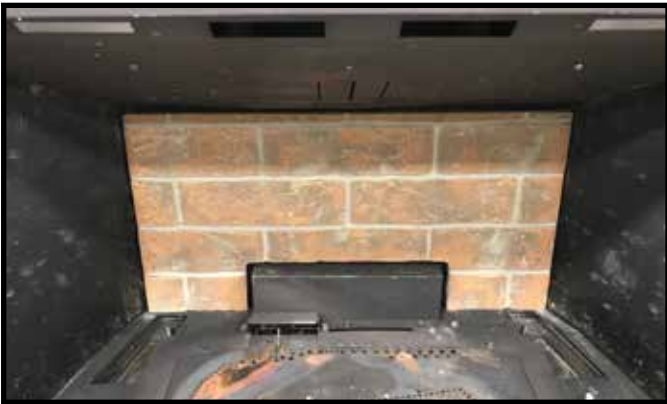
Figure 4 Back Refractory Installed
