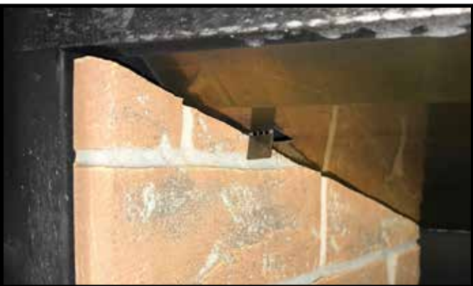
Figure 6 Left Refractory Handbend Tab
