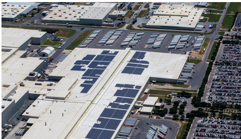
A 3.1 megawatt solar array was also installed on the roof of the assembly plant building. These panels are expected to generate around 3 percent of the plant's annual demand.
